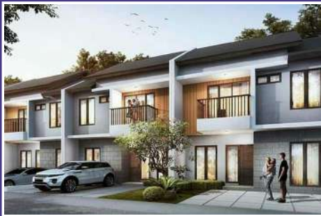
Asana Residence Cimanggis
